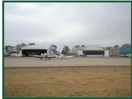
There is also a turf apron located west of the paved apron adjacent to the two connecting taxiways (see **Figure 2-3**). This apron is used for long-term aircraft parking and storage. This apron is approximately 25,000 square yards and has 17 aircraft tie-downs.
